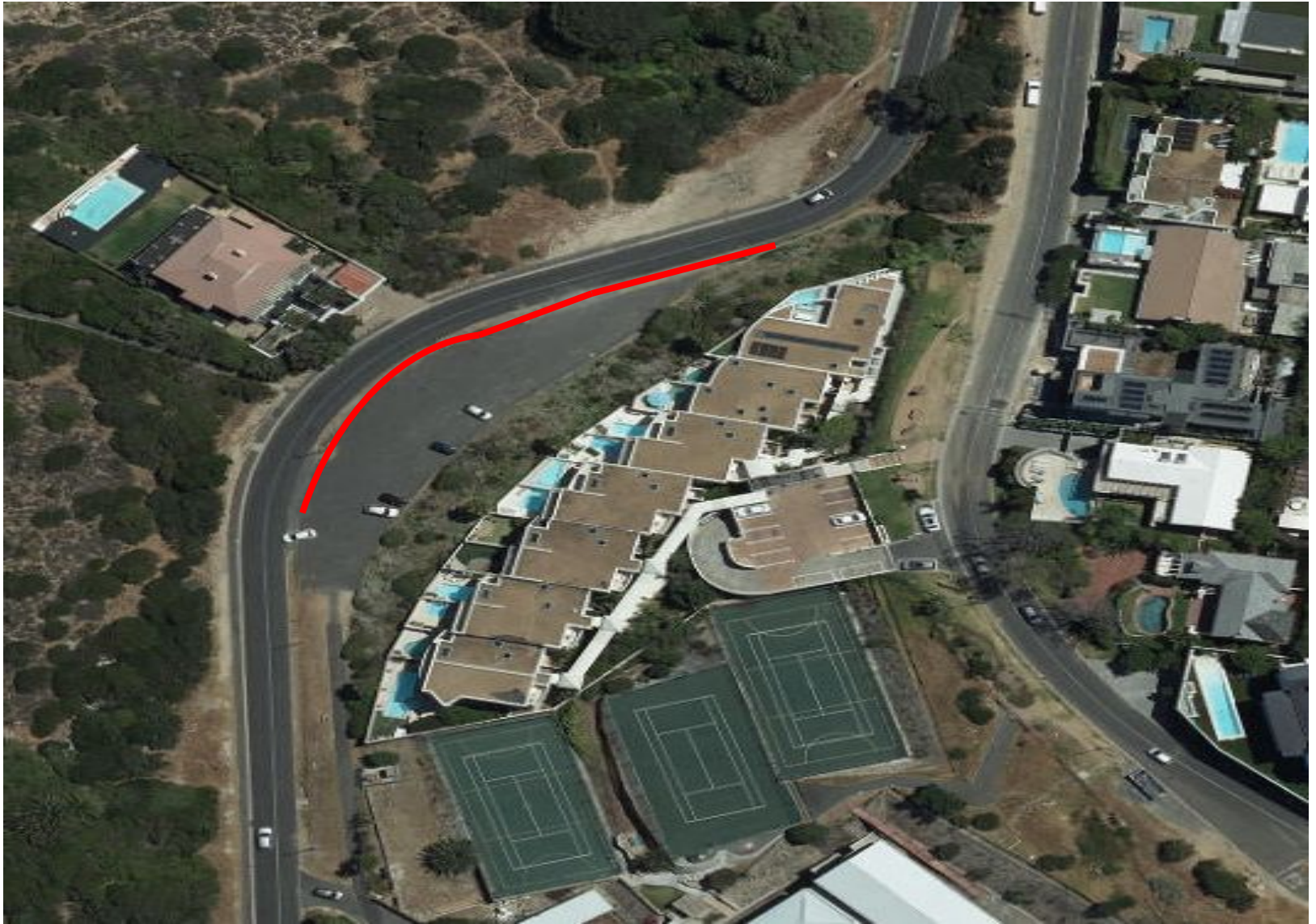
Kloof Rd, Parking lot fencing
